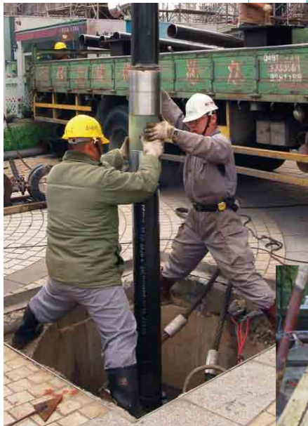
Hot spring well fix engineering
