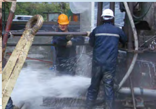
Hot spring well wash engineering
